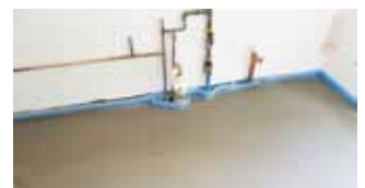
Minitec with screed applied
